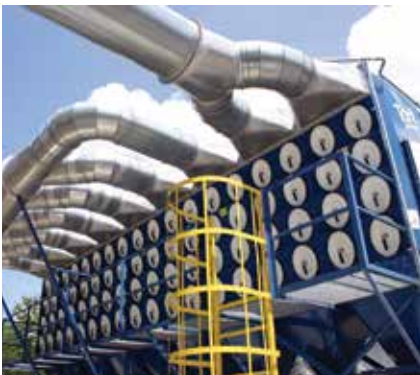
DFO on Sawdust 57,500 cfm (97,692 m 3 /h)
