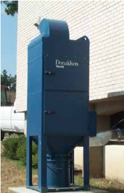
UMA - School Wood Shop 2,000 cfm (3,397 m 3 /h)
