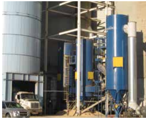
RF - Grain Terminal 34,000 cfm (57,754 m 3 /h)
