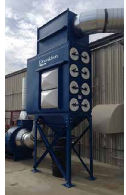
DFO on Plastics Routing 16,000 cfm (27,184 m 3 /h)
