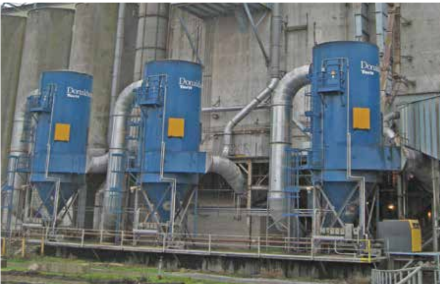
RF - Grain Terminal 61,000 cfm (103,618 m 3 /h)
