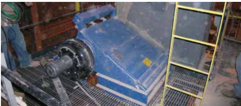
CPV - Bucket Elevator 1,200 cfm (2,038 m 3 /h)
