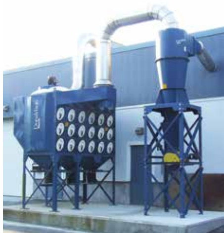
DFO & CYCLONE on Thermal Spray 4,800 cfm (8,154 m 3 /h)
